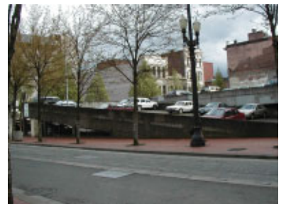
Not Recommended: Exposed sloped parking structure
