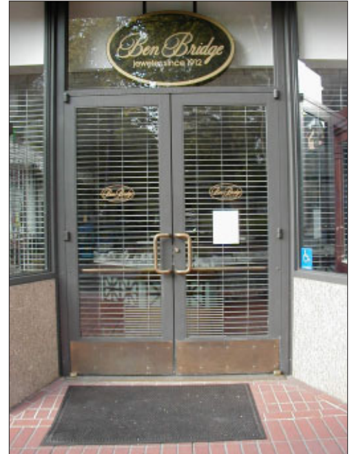
Appropriate: Interior, roll-up security gates.
