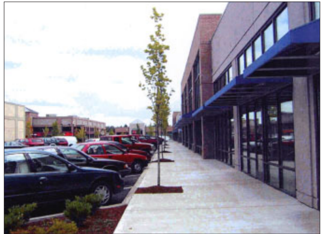
Inappropriate: Storefront windows without panels below
