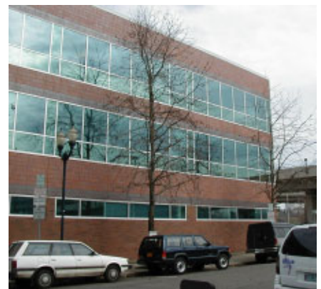
Inappropriate: Horizontal strip windows flush with building facade
