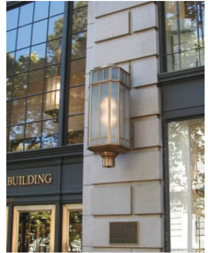
Recommended: Decorative wall sconce designed as part of overall building facade composition
