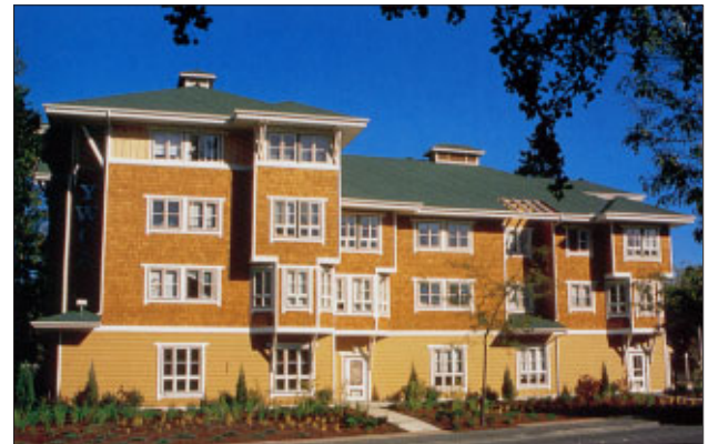
Appropriate: Boldly articulated facades benefit from the inclusion of medallions, belt courses, varied cladding materials or other surface articulation
