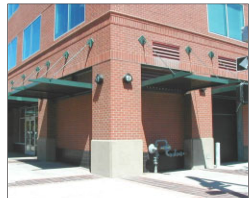
Inappropriate: Unwelcoming blank walls at building corner
