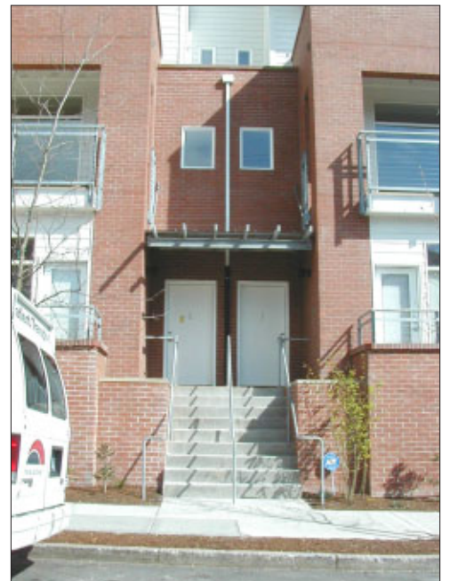
Inappropriate: Colorless and unarticulated entry doors do not convey a welcoming appearance
